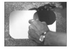
3. Install door in opening (insert at an angle).
