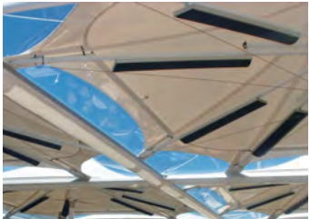
Roof Infills & Link Gutter detail
